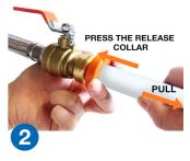
Step 2: Firmly push the removal tool over the collar of the fitting.
